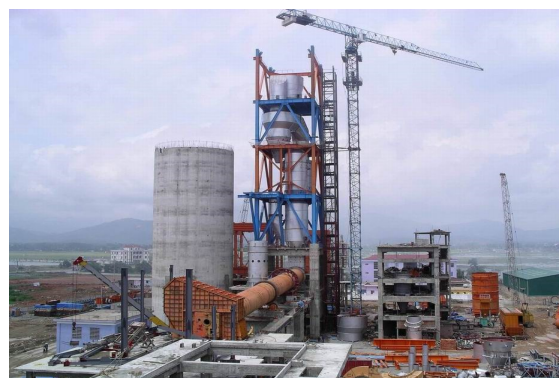
Lam Thach Cement Factory
