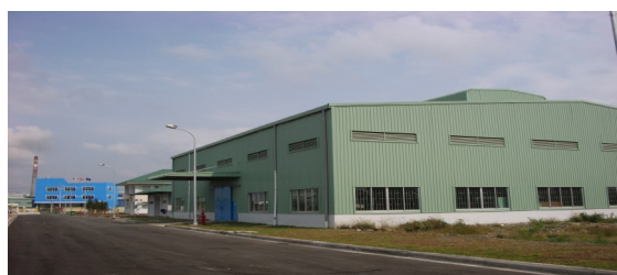
No.1 Cast Plant
